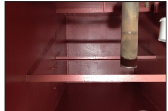
Completed tank internals
