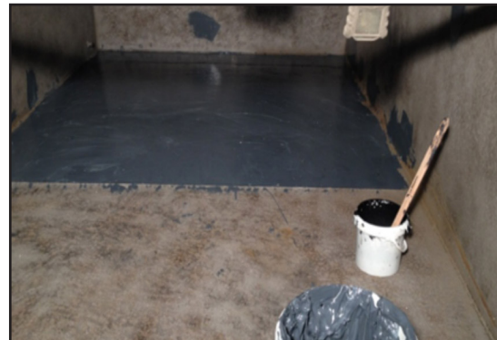
Applying ARC 858 to resurface and fare smooth pitted surface
